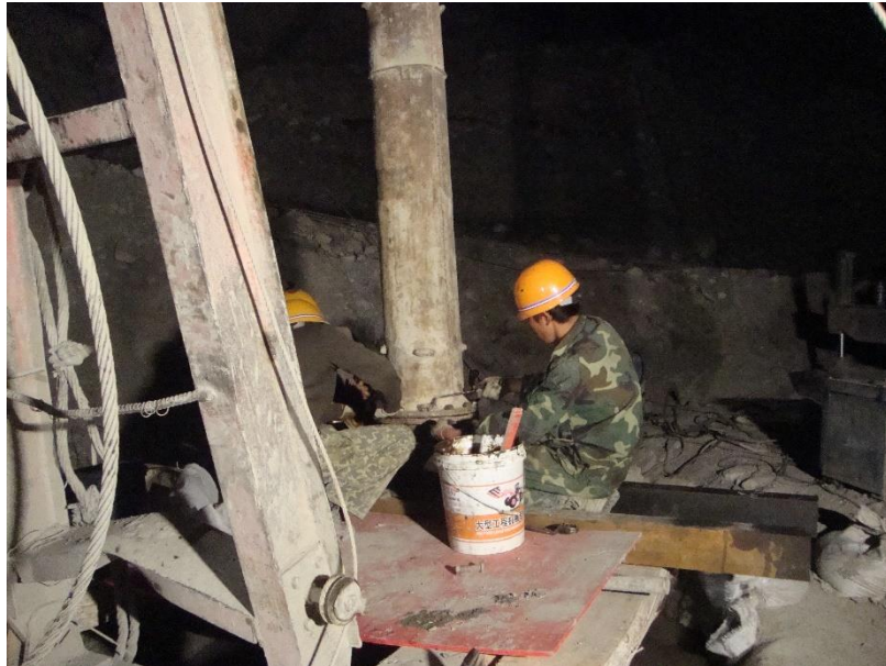
晚上加班冲孔 Overtime drilling at night
