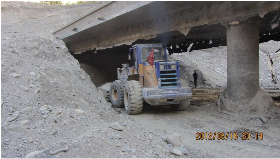
土台拆除现场（箱梁底板） Soil removal site (box girder floor)
